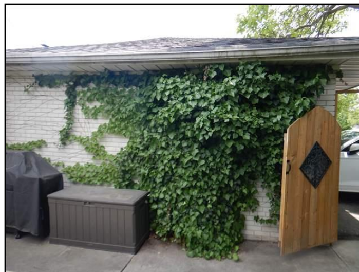
Vines on building
